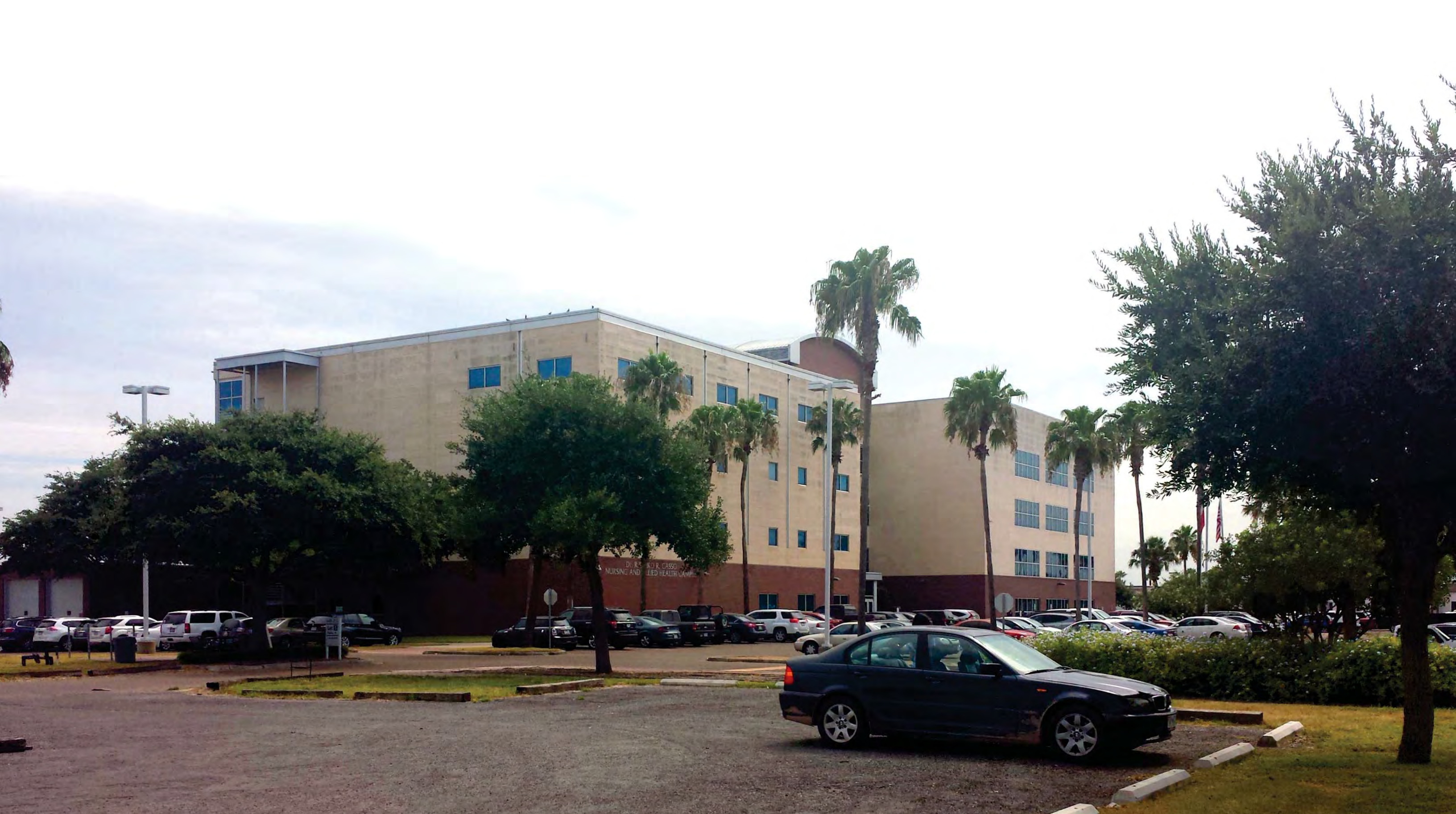
EXISTING SOUTH WEST VIEW
