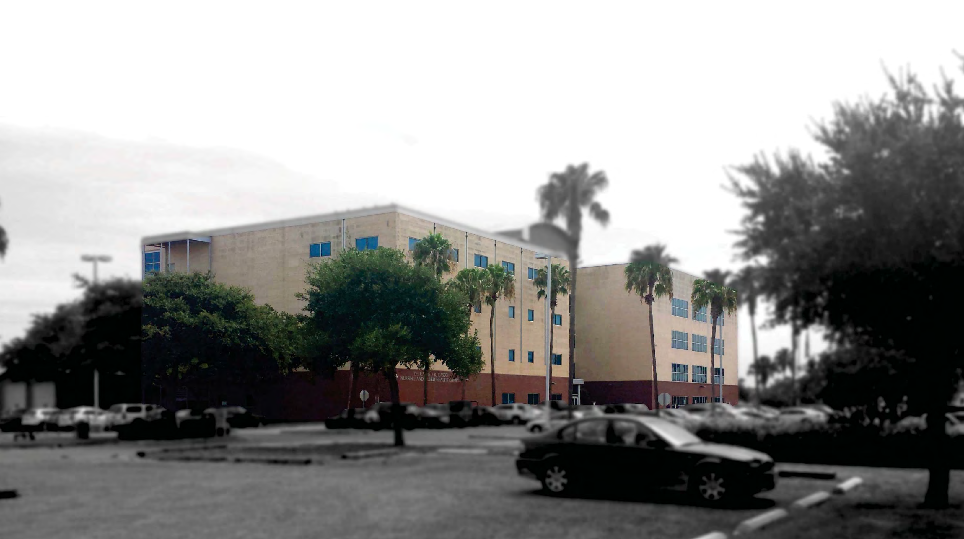
EXISTING SOUTH WEST VIEW
