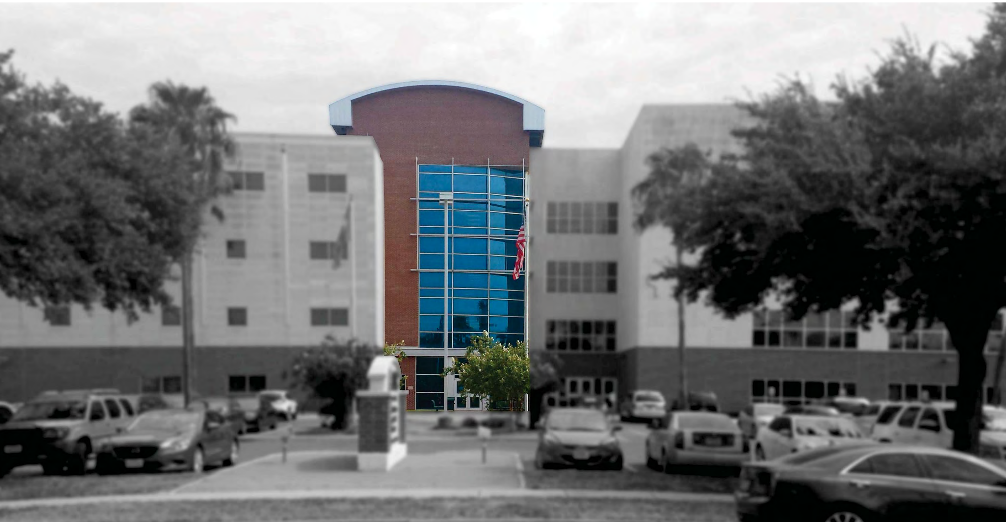
EXISTING SOUTH VIEW
