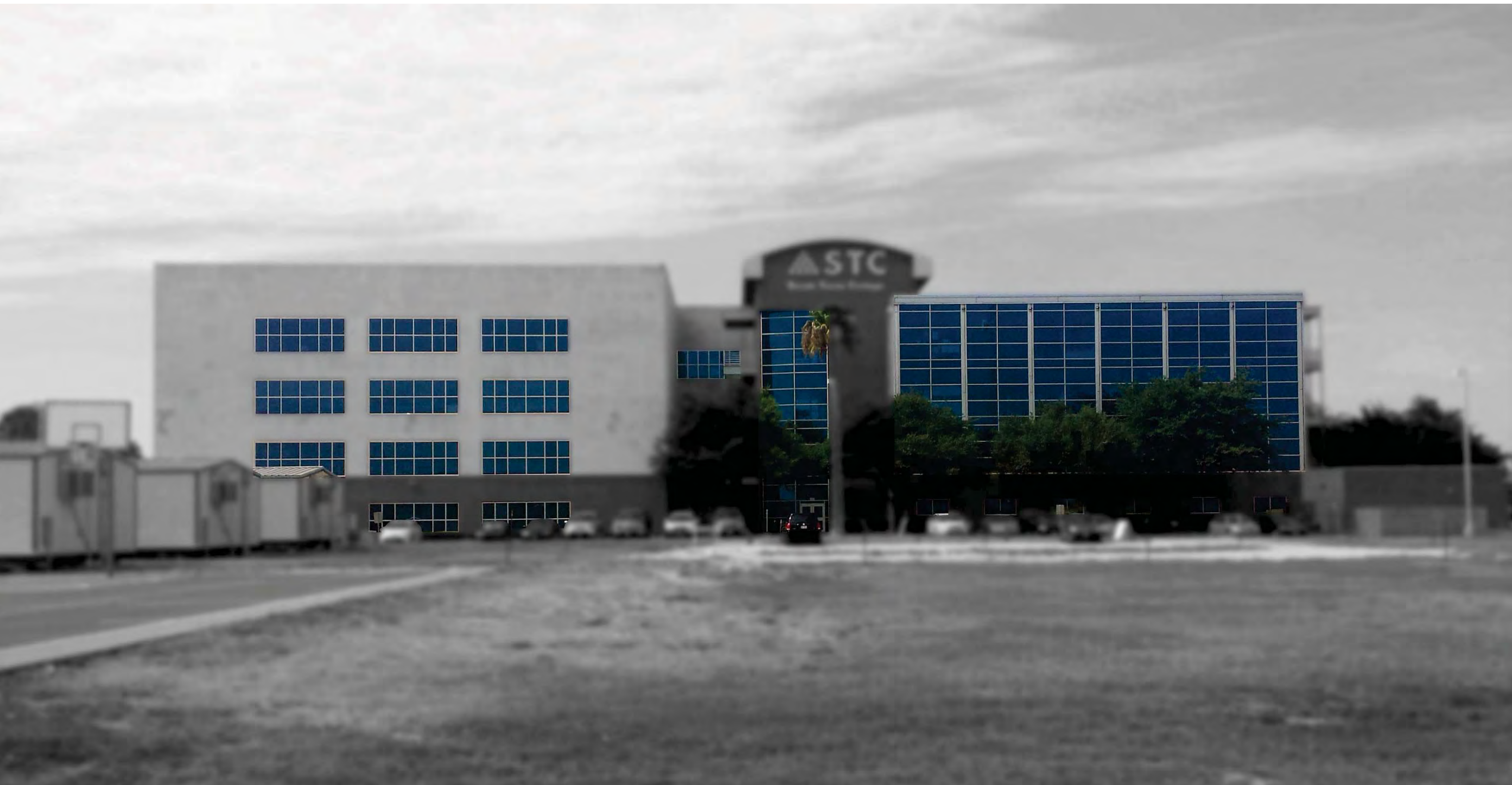
EXISTING NORTH VIEW
