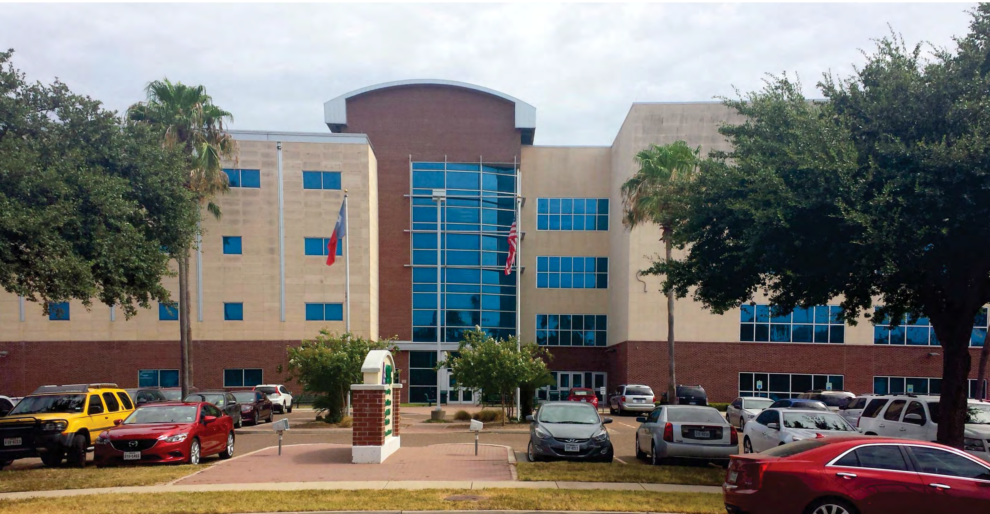
EXISTING SOUTH VIEW
