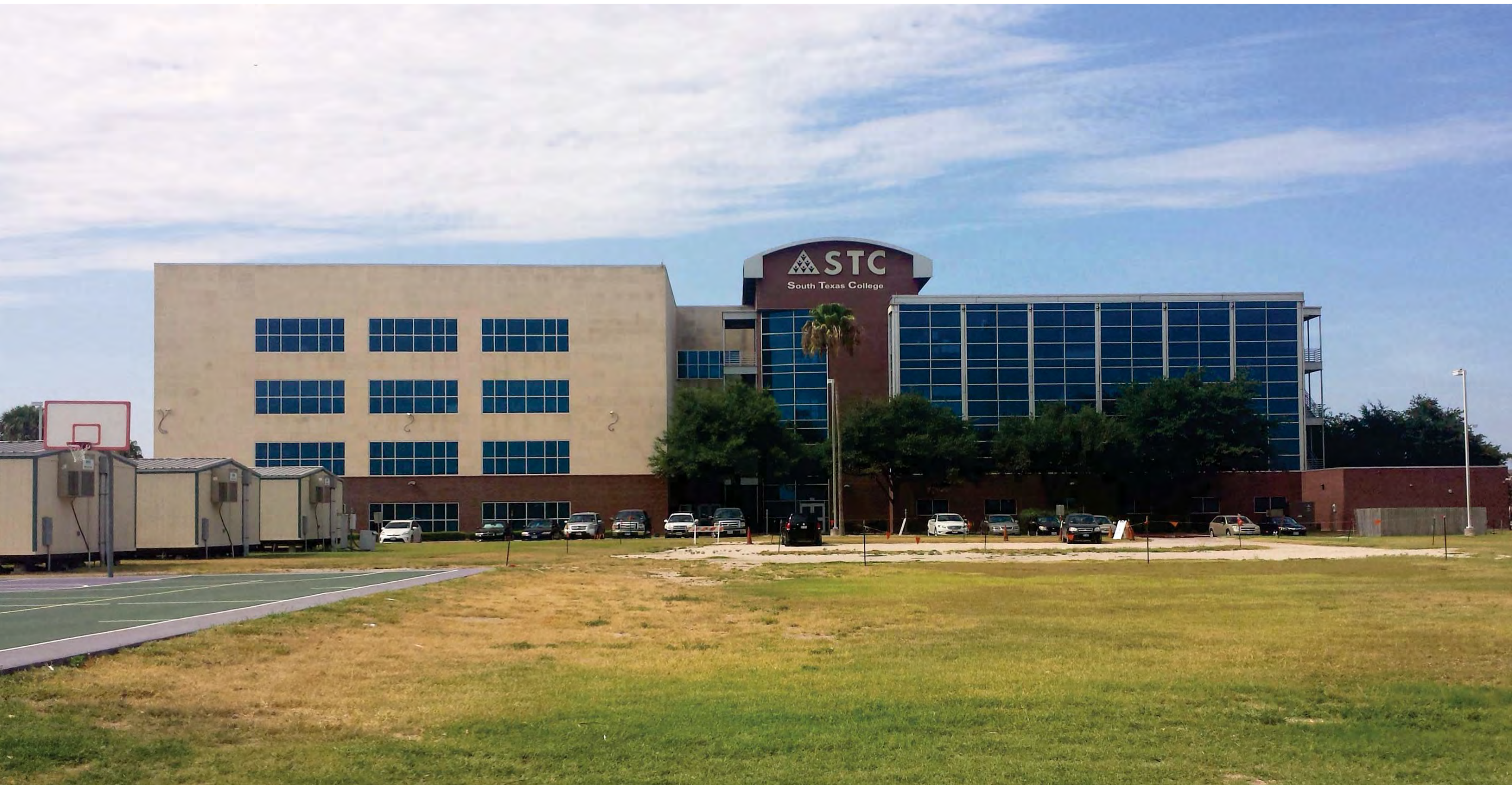
EXISTING NORTH VIEW
